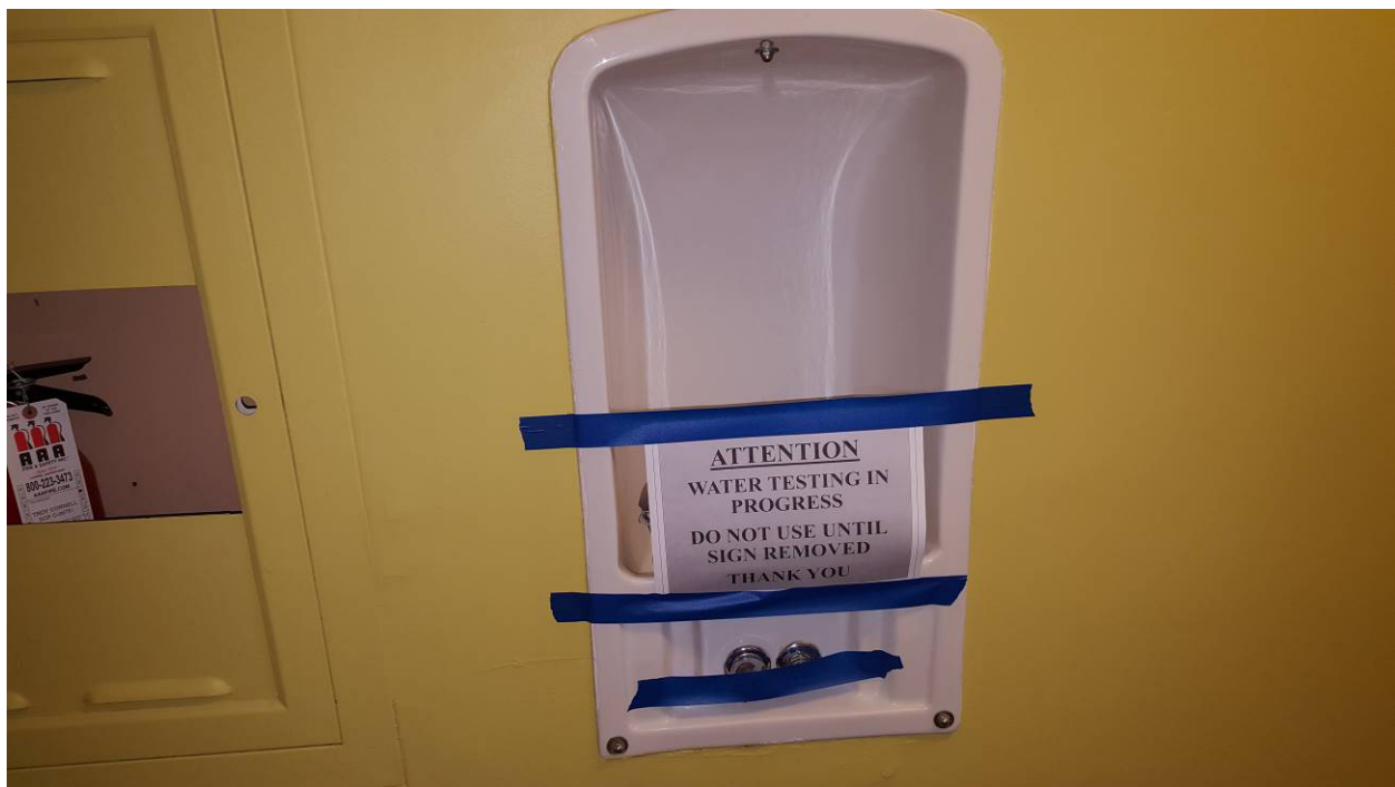
Photo 2, Example of water testing sign on recessed wall mounted bubbler
