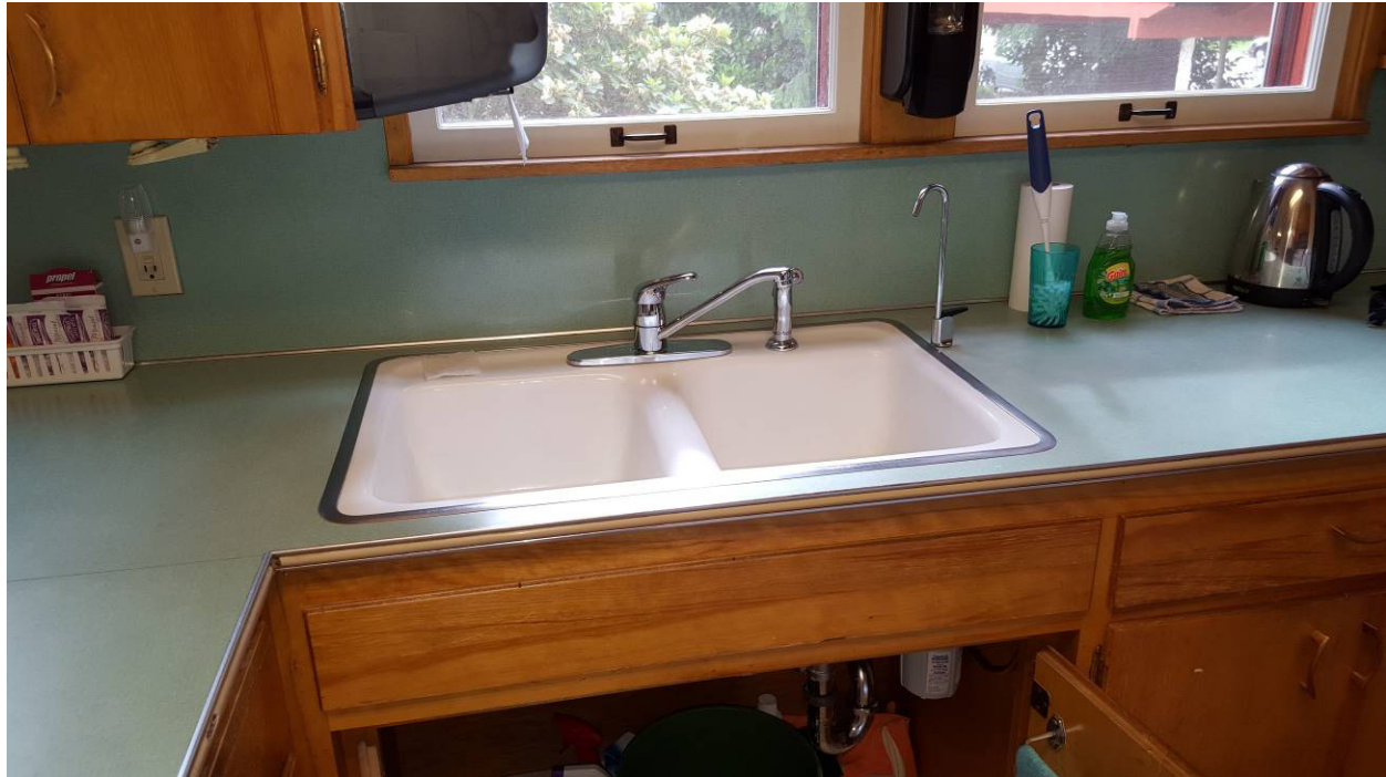
Photo 3, Payroll House kitchen sink faucet with filtered bottle filler, Sample FD-19
