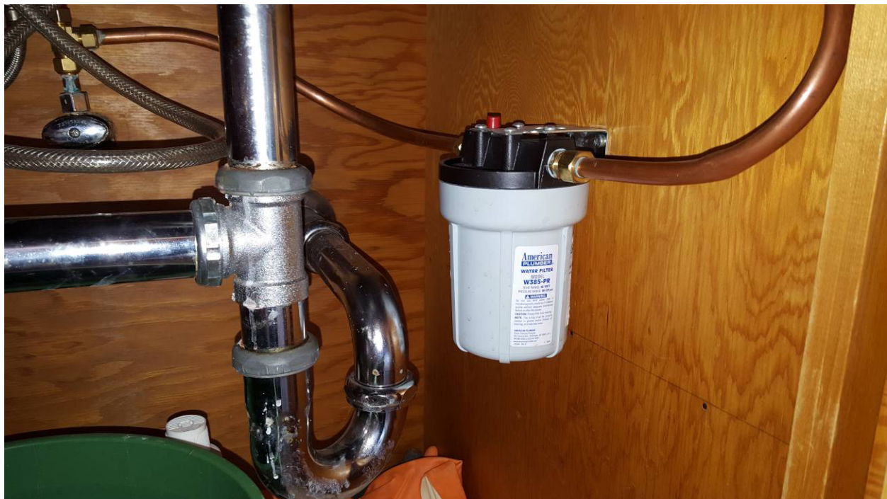
Photo 4, Payroll House kitchen sink water filter in cabinet below sink
