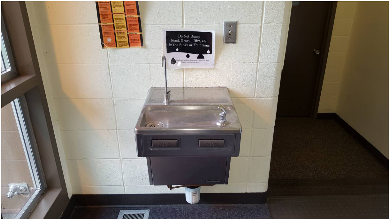
Photo 8, Pflueger Hall 1 st floor lobby, wall mounted water cooler with filtered bottle filler, Sample FD-31
