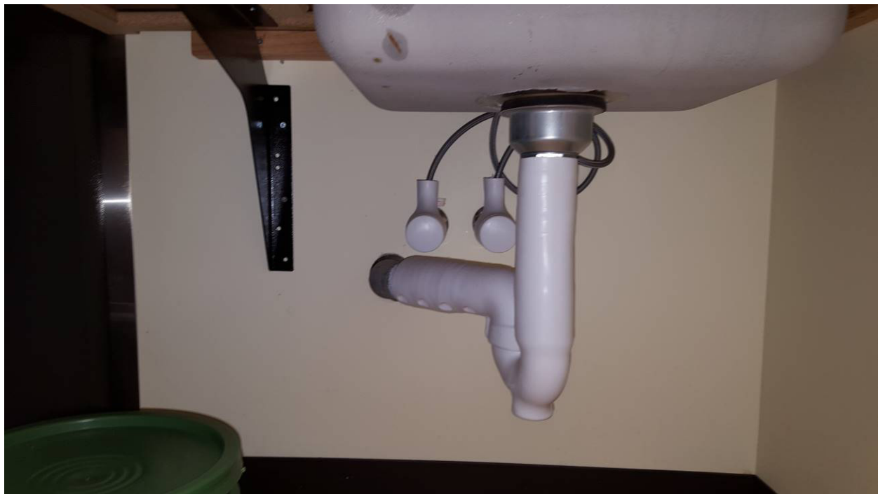
Photo 6, Stuen Hall Room 303, unfiltered water lines below sink
