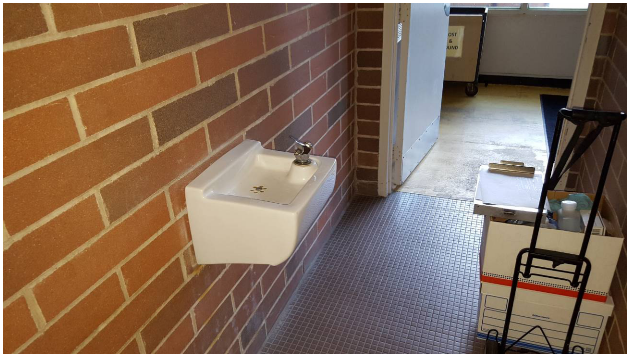
Photo 14, Swimming Pool, unfiltered wall mounted ceramic bubbler, Sample FD-40
