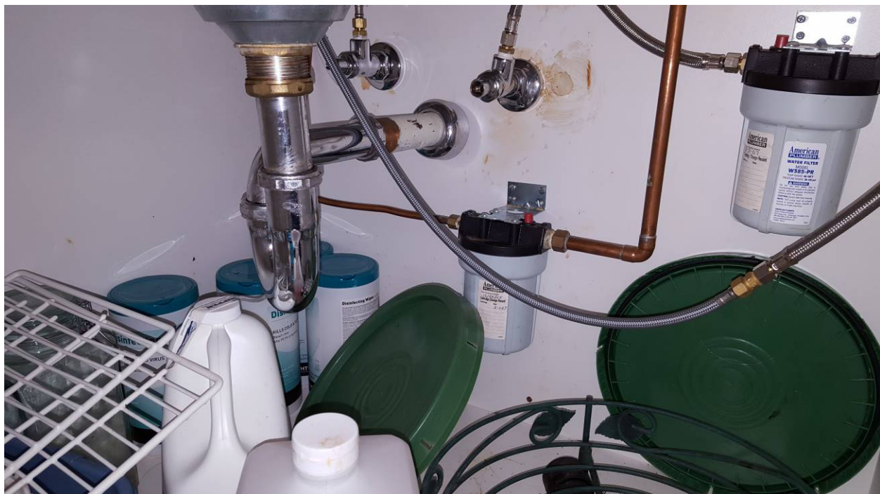
Photo 12, Morken Center School of Business staff break room, water filters for faucet and coffee pot in cabinet under sink
