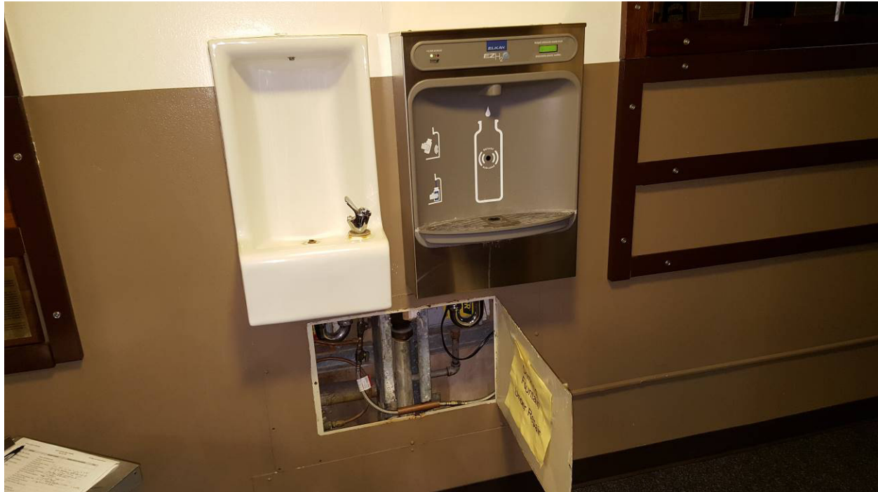
Photo 13, Olson Auditorium, wall mounted unfiltered bubbler next to wall mounted filtered bottle filler, Sample FD-47 taken from bottle filler
