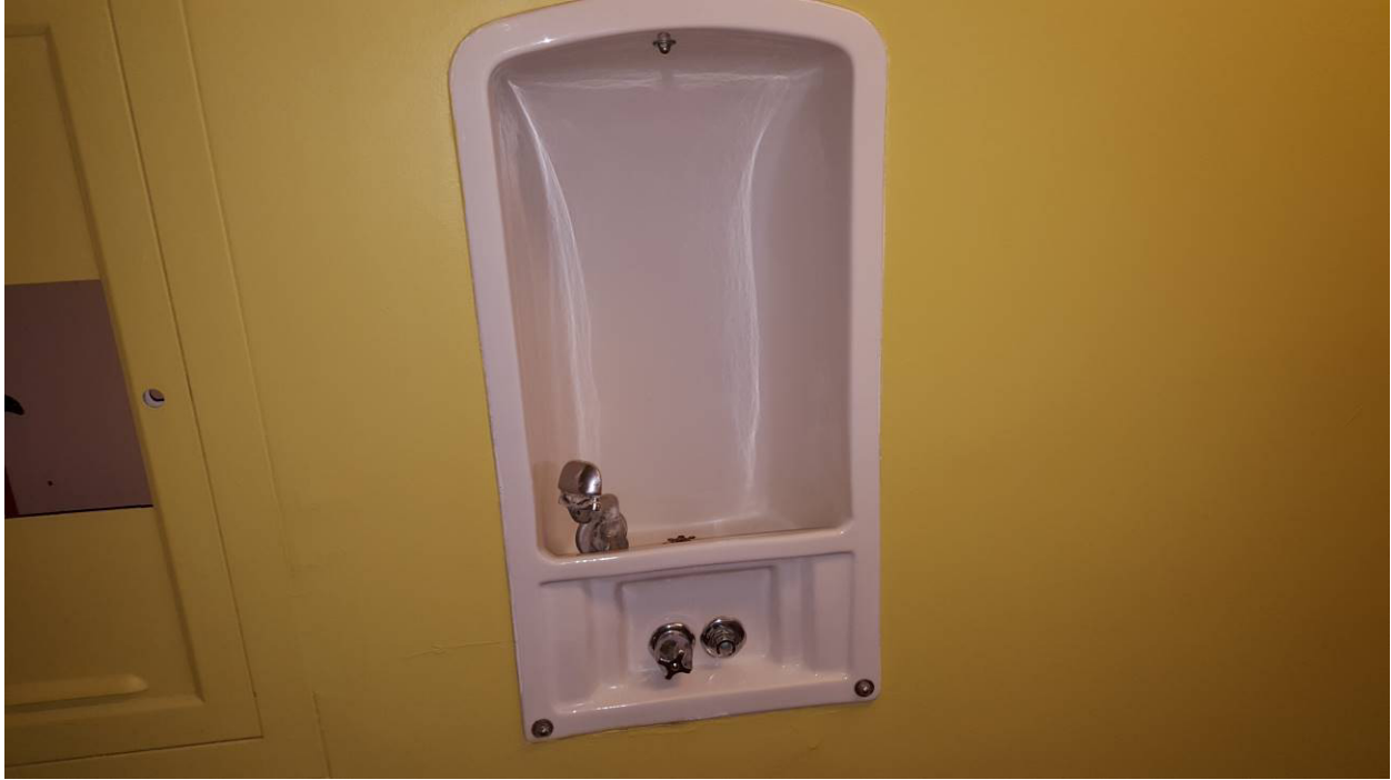
Photo 15, Hong Hall, 3 rd floor, recessed unfiltered ceramic bubbler, Sample FD-60
