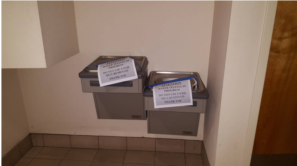
Photo 9, South Hall 1 st floor by N entry, dual bubbler without bottle filler, Sample FD-26 taken from upper bubbler
