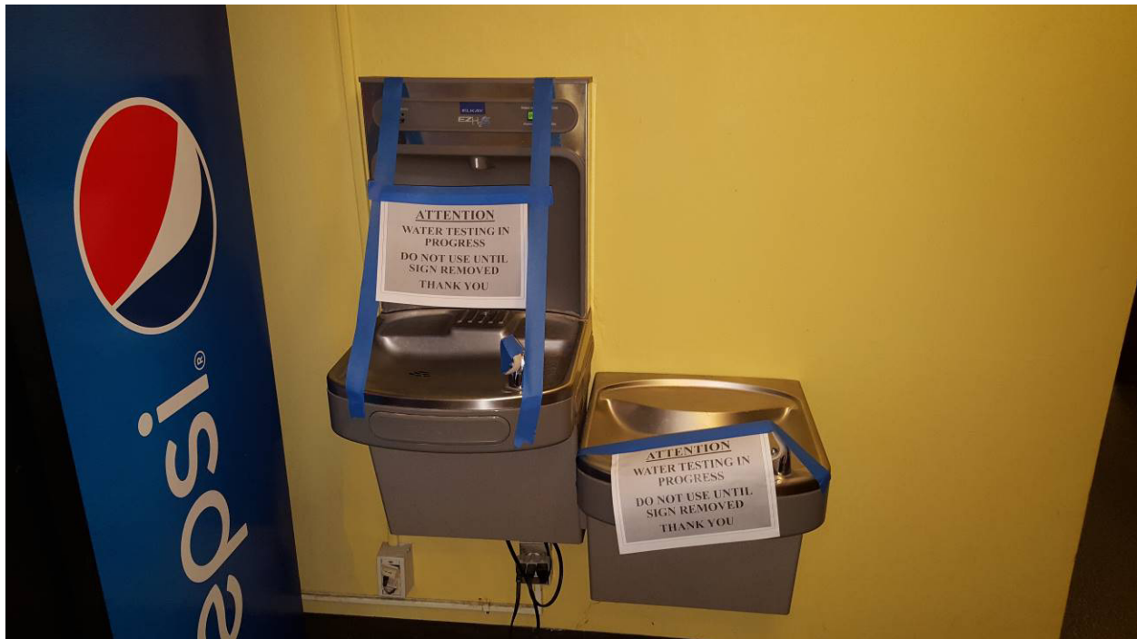
Photo 1, Example of water testing signs placed on dual bubbler with bottle filler
