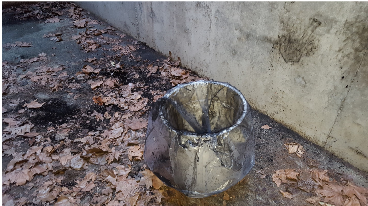
Photo 6, Soot residue after cleaning vacuum filters
