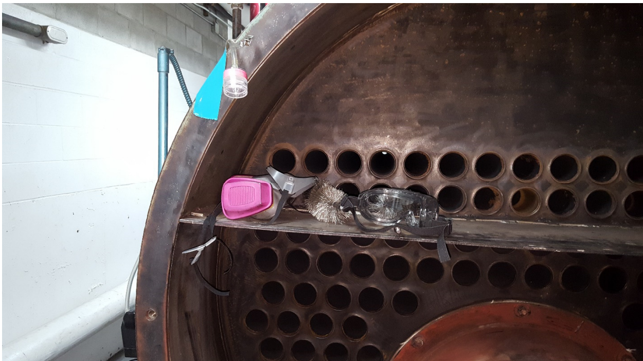
Photo 12, Respirator and safety goggles left on boiler during break.
