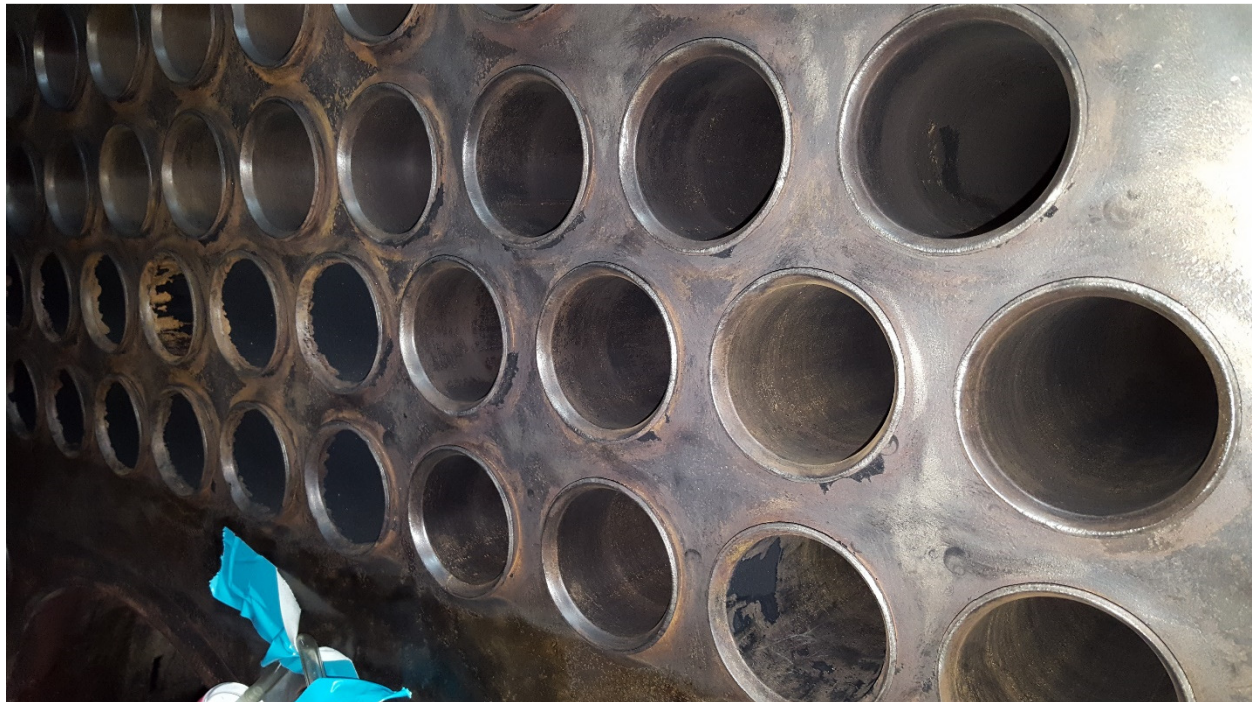
Photo 9, Wider view of small fire-tubes after cleaning
