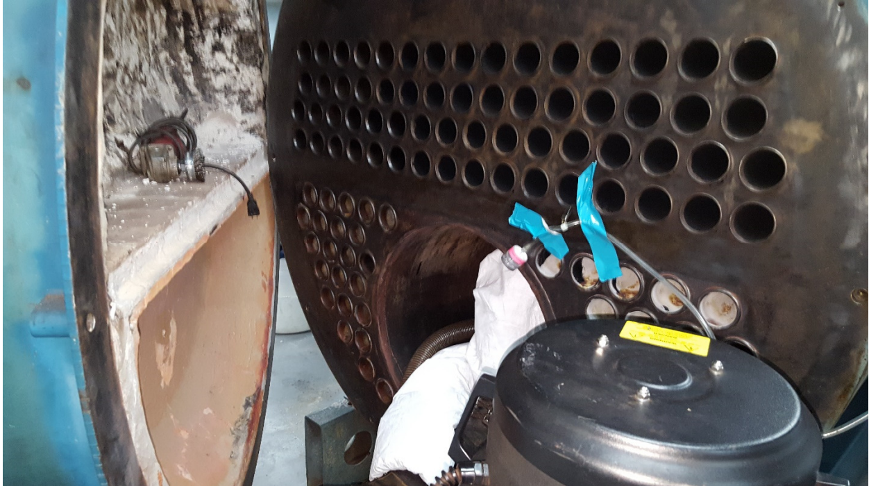
Photo 1, Cleaning Morrison tube. Area total dust sample is just above vacuum.
