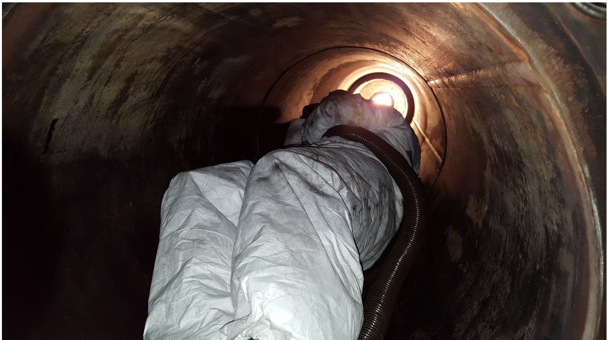
Photo 2, Employee inside Morrison tube, cleaning with electric brush and vacuum.
