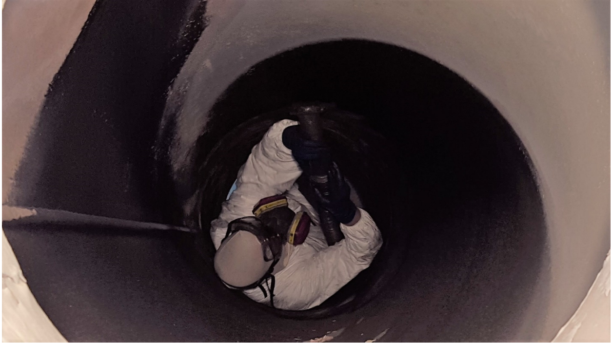
Photo 3, View of Morrison tube cleaning from burner side of boiler,
