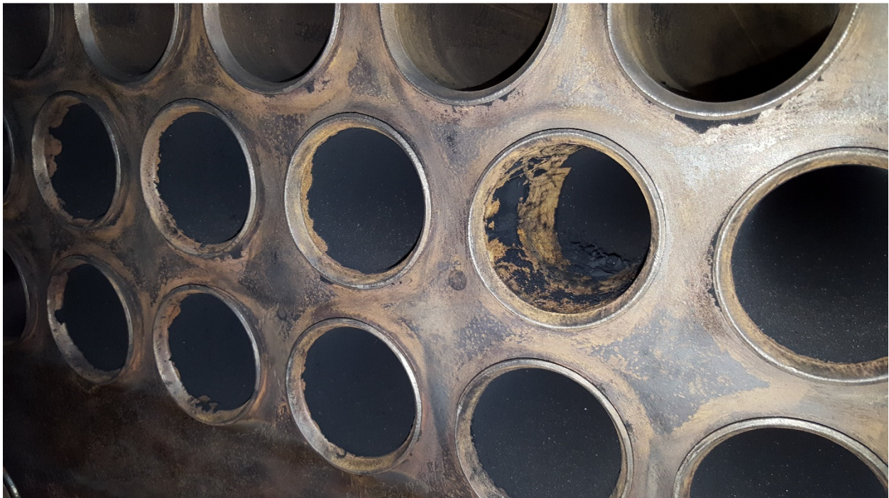
Photo 8, Soot buildup in small fire-tubes before cleaning. Top row has been cleaned.
