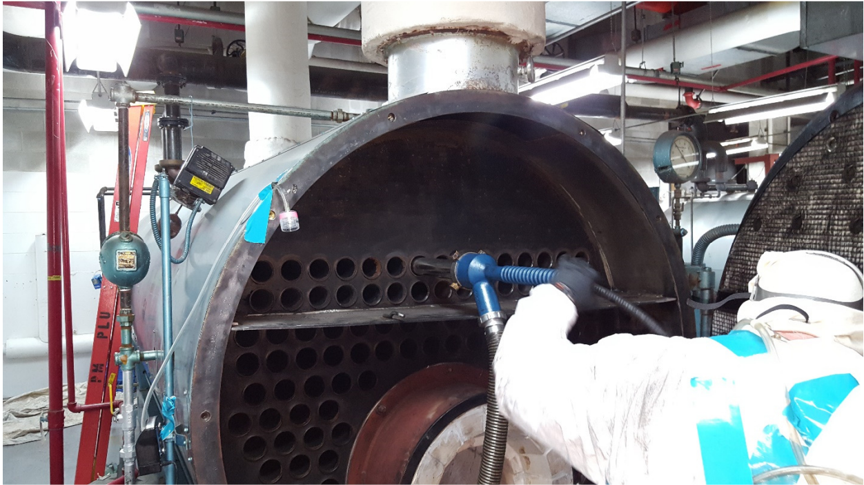
Photo 7, Cleaning upper fire tubes with brush and vacuum system while wearing air sampler for PAHs. Area total dust air sample on upper left side of boiler.
