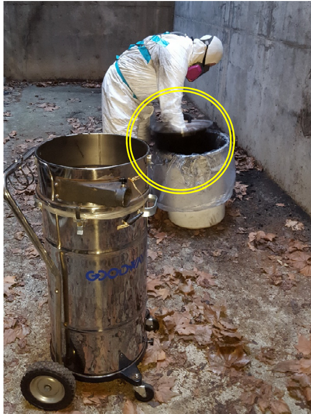
Photo 5, Dust released by shaking Soot Vac filter to remove soot.
